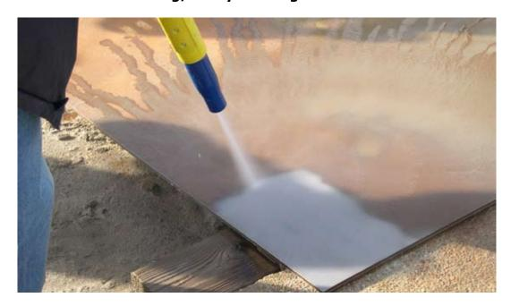
Wet abrasive blasting uses a slurry of water and abrasive rather than dry abrasive alone. This has the advantage that the hazards of dust and associated health problems are largely overcome.
